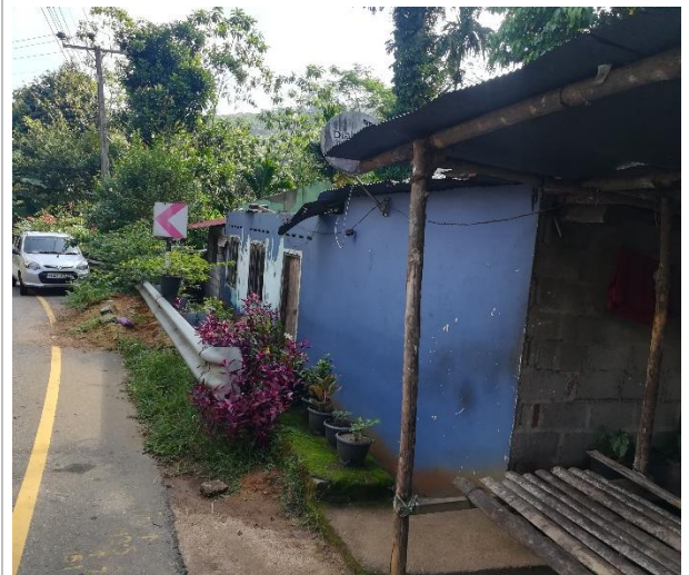
Figure 05 (b) – House locate at the potential slope failure location is prepared to move safer location.
