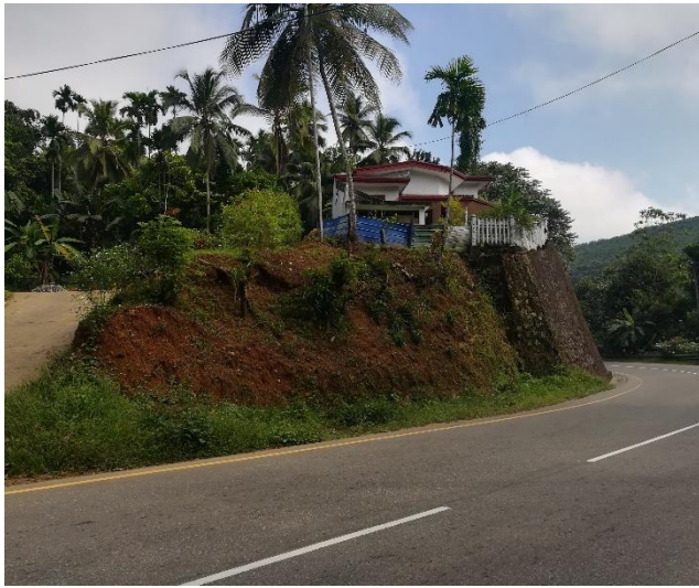
Figure 05 (c) – Location of house with retaining wall adjacent to landslide mitigation site.
